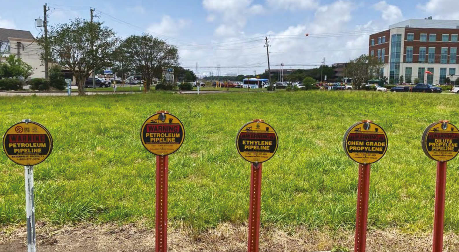
Petroleum and petrochemical pipelines run alongside a hospital in Baytown, Texas, © Amnesty International, May 2023
