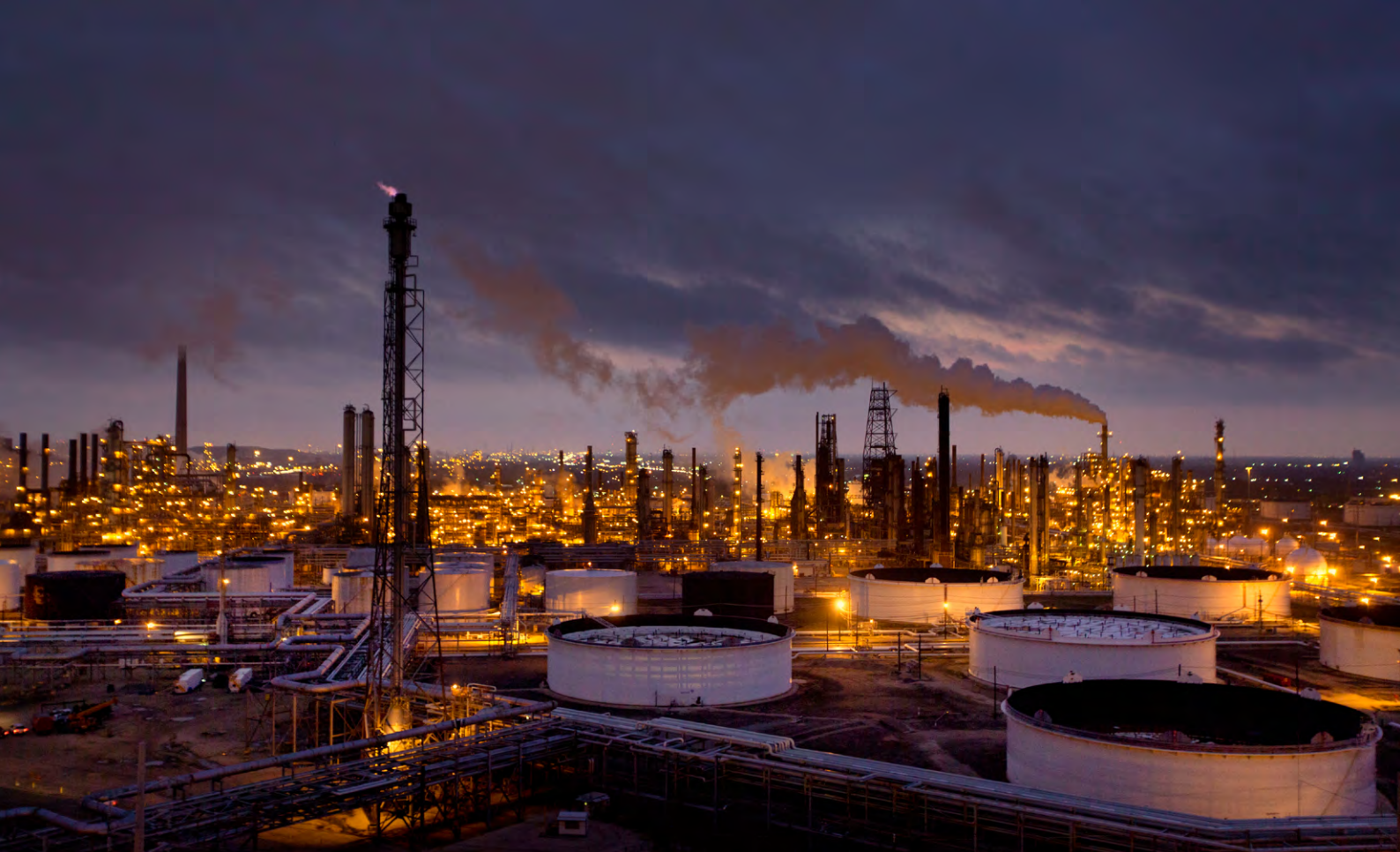
Petrochemical plants along the Houston Ship Channel. © Getty Images (Photographer: Ed Lallo)
