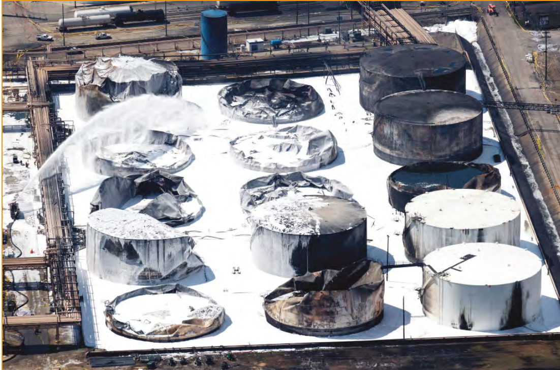
Emergency crews extinguishing the petrochemical tank fire at ITC Deer Park with firefighting foam. The fire began on 17 March 2019 and lasted over three days. © 2019 Houston Chronicle via Getty Images (Photographer: Brett Coomer)
