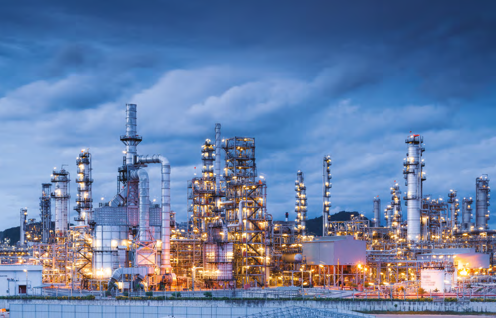
A petrochemical plant lit up at night. © Getty Images (Photographer: Chanin Nont)
