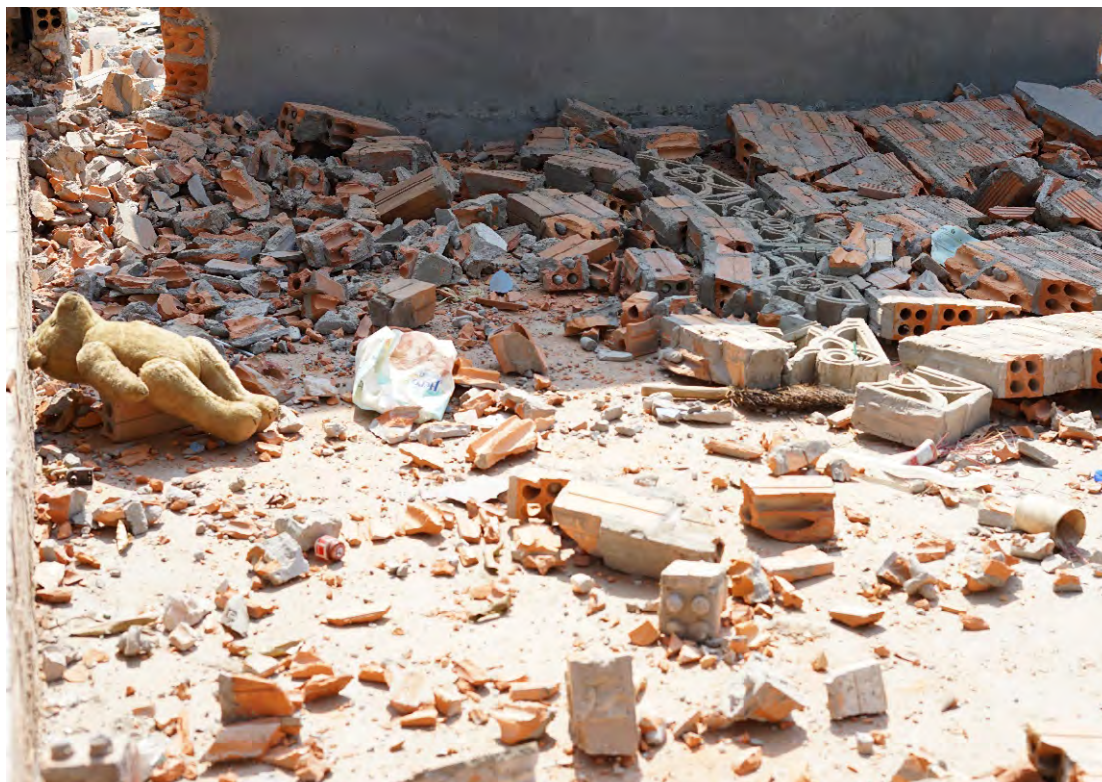
A teddy bear amongst the rubble of a house at Angkor World Heritage Site, March 2023, Amnesty International.
